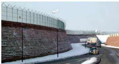
Paris Orly Airport (94), France
